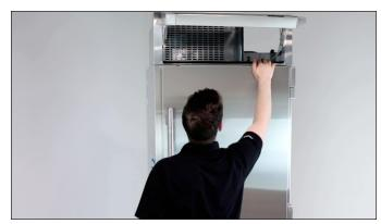
FIG. 3. Be sure to inspect behind the rainshield.
