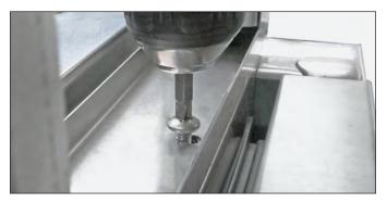
FIG. 10. Remove the screws from the metal channel.
