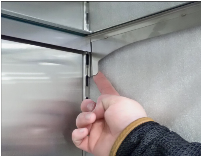
FIG. 6. Push the bottom tab inward.
