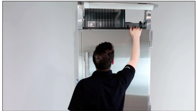
FIG. 3. Be sure to inspect behind the rainshield.
