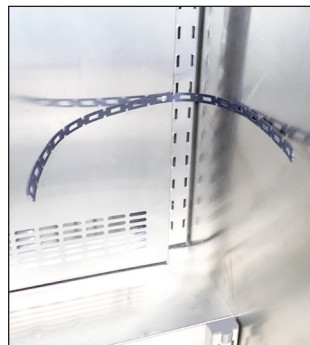
FIG. 8. Installed safety strap.
