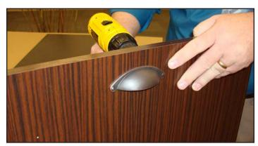
Image 4. Attach drawer handle to overlay panel.
