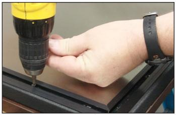
Image 9. Anchor overlay on door front.
