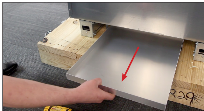
FIG. 9. Remove the drain pan before pulling the appliance off the skid.
