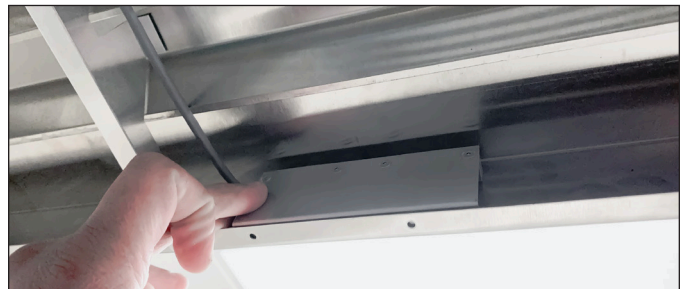
FIG. 3. Locate the reed switch in the bottom of the rainshield.
