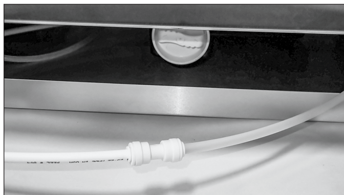
FIG. 1. Water line connection. Fitting included, PEX not included
