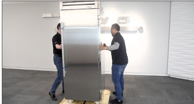
FIG. 11a. With assistance, carefully walk the appliance partially off the back of the skid.
