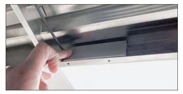
FIG. 3. Locate the reed switch in the bottom of the rainshield.
