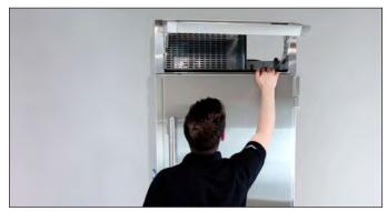
FIG. 3. Be sure to inspect the rainshield.
