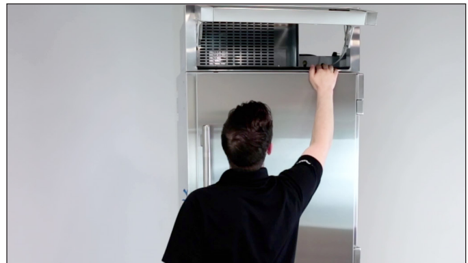
FIG. 3. Be sure to inspect behind the rainshield.
